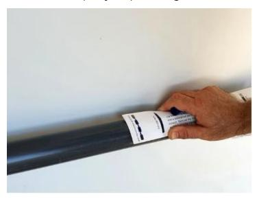
2. Using a hack saw, cut the pipe in the marked location.
